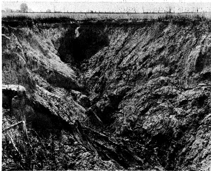
W. F. PURNELL FIG. 3 — GULLY EROSION PRODUCED BY THE CONCENTRATION OF WATER IN THE NATURAL DRAINAGE WAYS OF A FIELD
