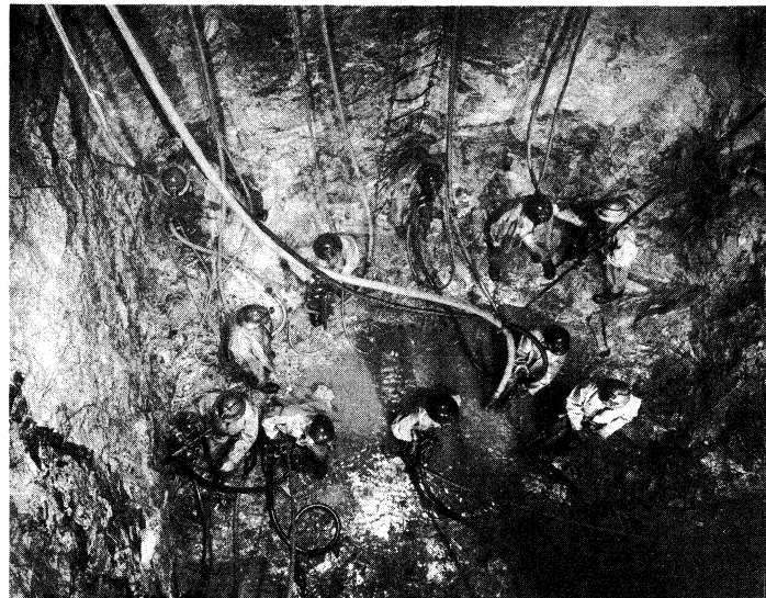
FIG. 4.— DRILLINGBY SHAFT-SINKING CREW
